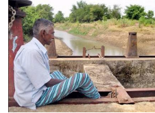
Sluice gate closure at Mavil Aru
