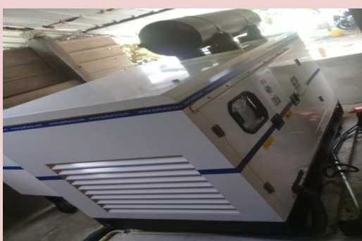
Installation and commissioning of 30 KVA Generator at CGS 'Panadura'.
