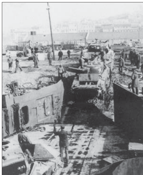
A US M-4 Sherman tank pushes another Sherman tank onto a Landing Ship Tank (LST) at Inchon for evacuation to Japan and repair. In the Marine 1st Tank Battalion, Sherman tanks were used as flamethrower tanks and as dozer tanks because those capabilities had not yet been adapted to the M-26. (US Navy)
